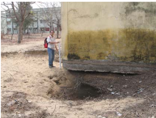
Figure 5-1. Tsunami Scour. Tsunami runup height = 4.1 m, Inundation depth = 0.95m above the floor; Scour depth = 1.2m. Photo provided by Harry Yeh.
