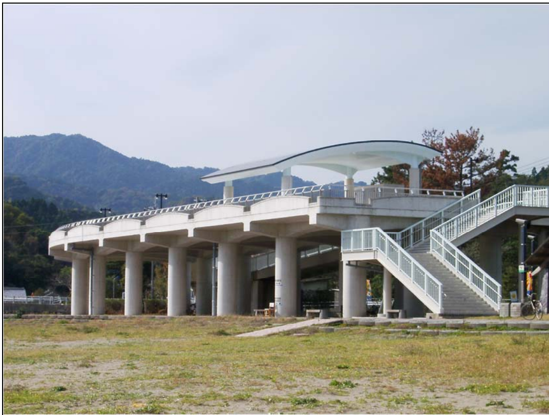
Shirahama Tsunami Evacuation Structure. Photo by Professor Nobuo Shuto
