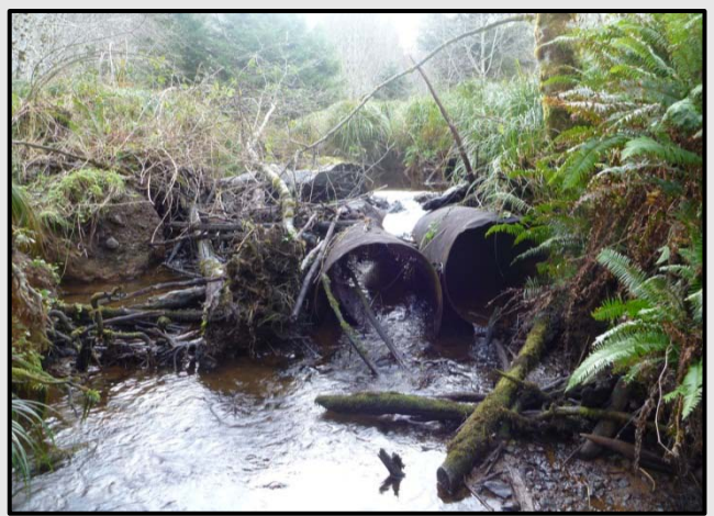
Remnant double culvert on Waterhouse Creek, a fish-passage barrier.
