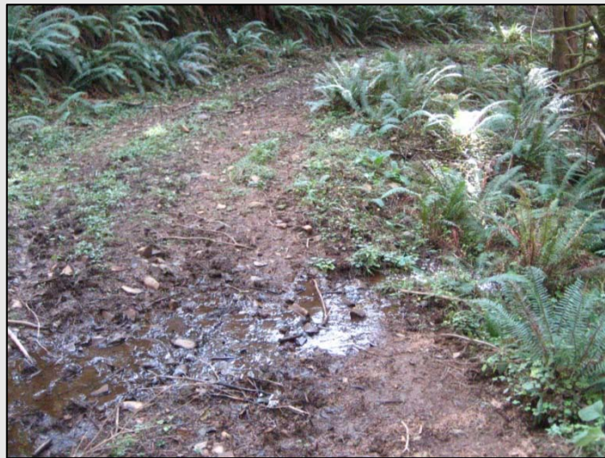
A plugged cross-drain culvert allowing water to cross a road surface in the NE part of ECFR.
